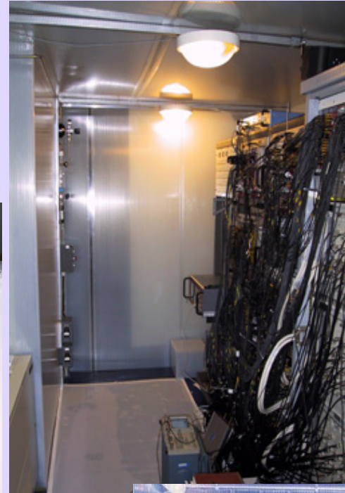
view with shielding completed
